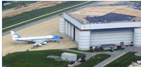
USAF - Joint Base Andrews Gate Improvements
