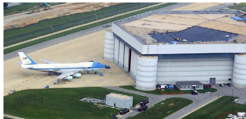
USAF - Joint Base Andrews Gate Improvements
